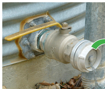
Figure 6 Ball Valve 65mm Storz fitting
